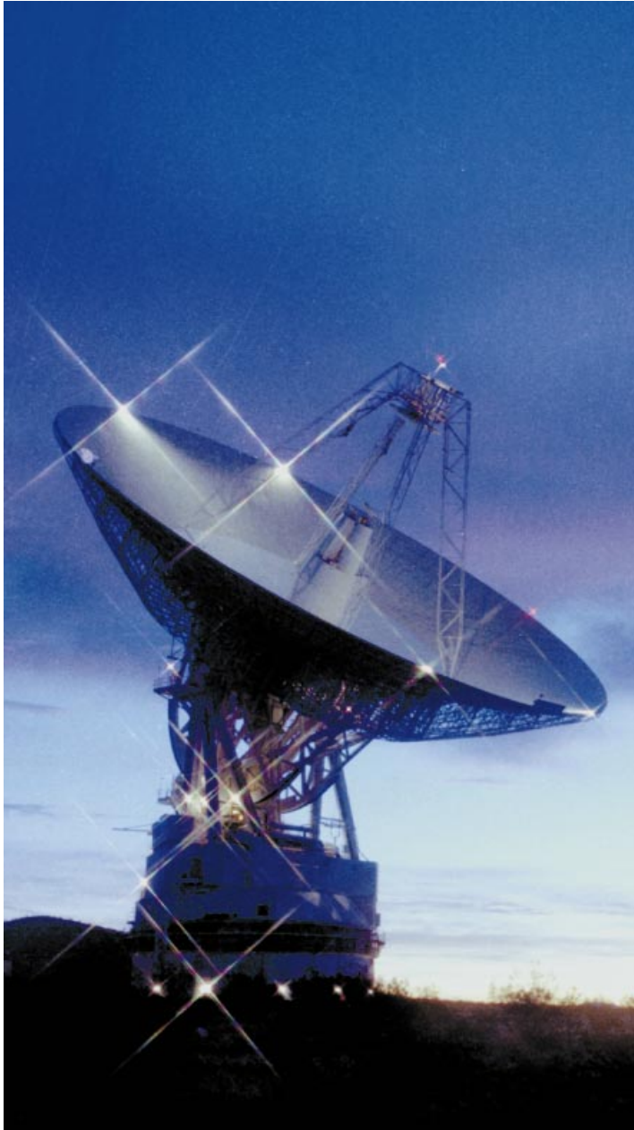
Figure 5. Exploration of the solar system depends critically on the worldwide collection of tracking antennas known as the Deep Space Network. The largest DSN antennas, like this 70-m-wide dish located northwest of Barstow, California, can receive transmissions from distant spacecraft far weaker than one-billionth of a watt.
